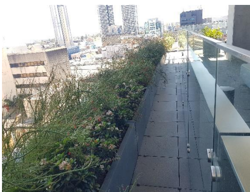
Figure 12: Level 6 Balcony Area – Steel capping provided to glass barrier to facilitate industrial rope access for façade and planter box maintenance.
