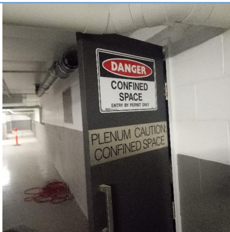
Photo 1. Lower Ground Car Park – Air Plenum observed to be incorrectly labelled as a confined space.
