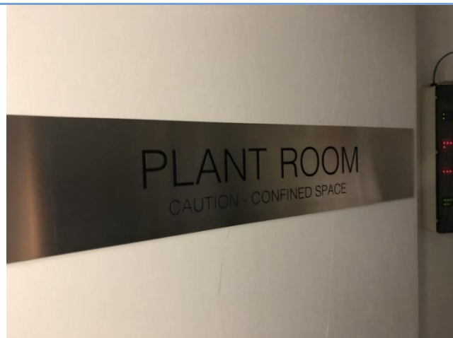
Photo 2. Ground Floor – Plant Room observed to be incorrectly labelled as a confined space.
