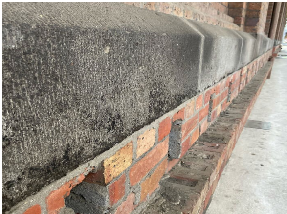
15. External east wall, bottom of stone course - Asbestos - Negative
