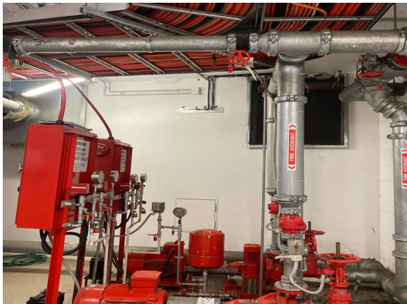
9. Fire Pump Room, back wall - Asbestos - Negative
