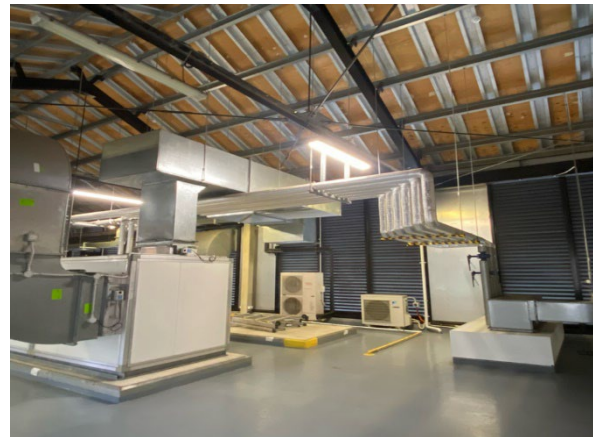
12. First Floor, Plant Room - Asbestos - Negative
