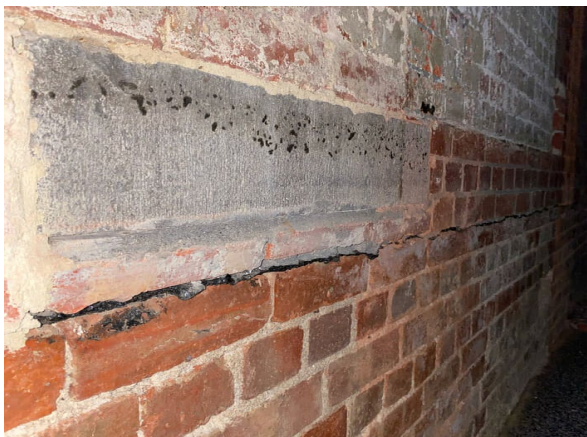
11. Central, dividing brick wall, damp proof course - Asbestos - Negative
