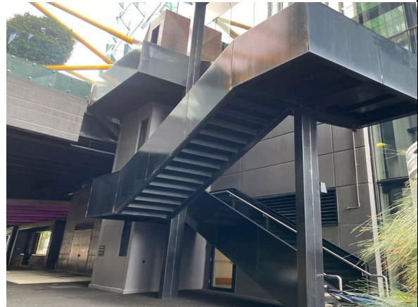
14. External stairs to upper level, wall panels - Asbestos - Negative
