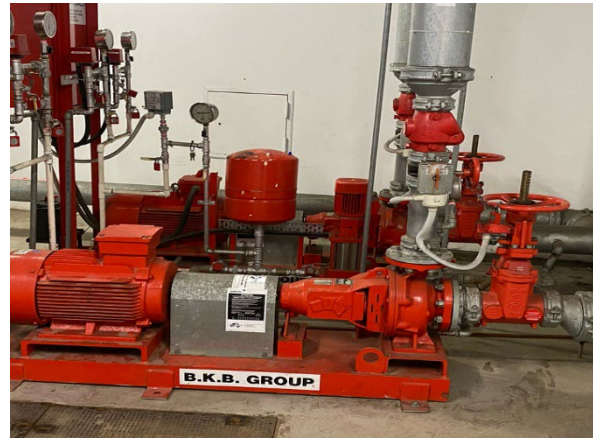
8. Fire Pump Room, pumps - Asbestos - Negative
